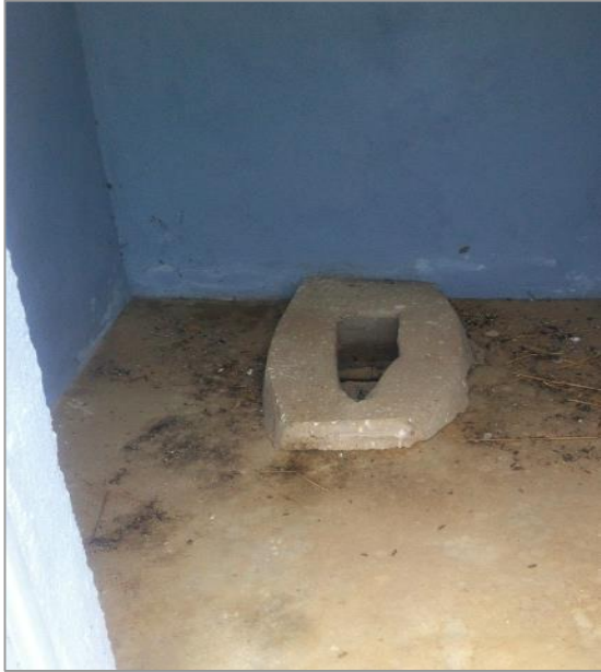
Concrete covering latrine
