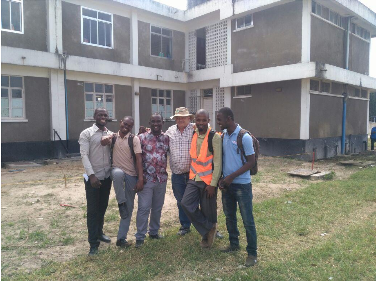
The picture shows the construction team. The yellow line behind the group is the reference line spanned across the future building site. The stick on the left marks the center of the digester to be constructed.
