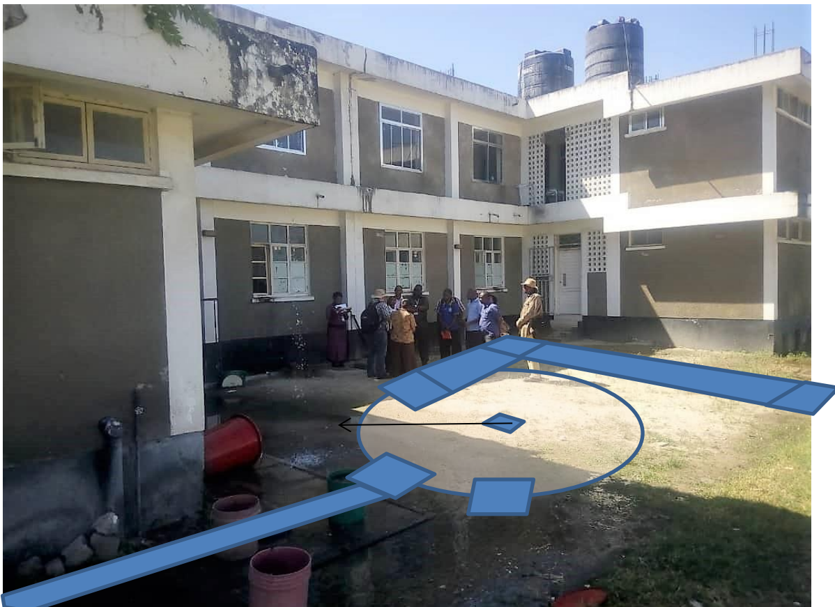
The site for construction was set out and marked on the ground
