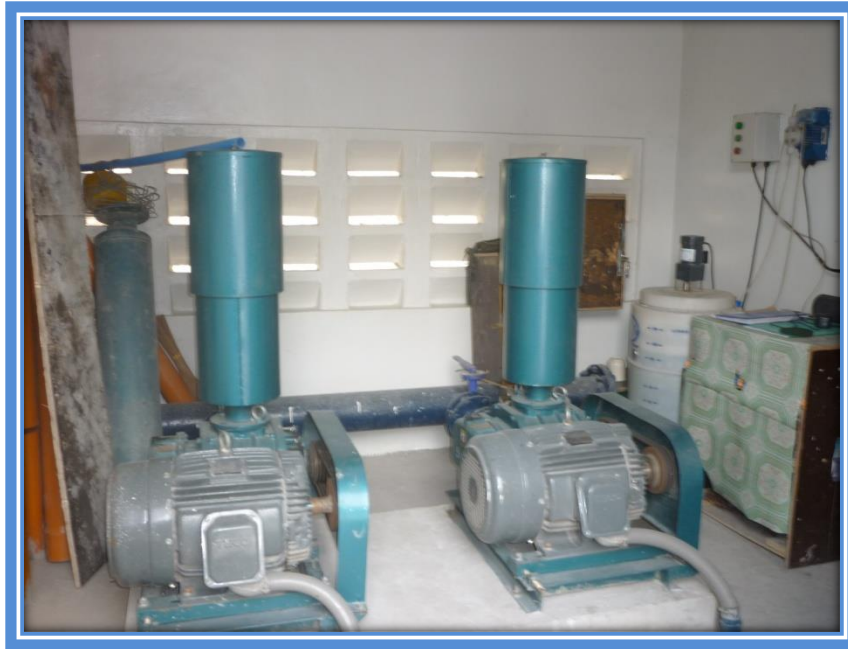
Figure 17- Wastewater Treatment Plant Facility
