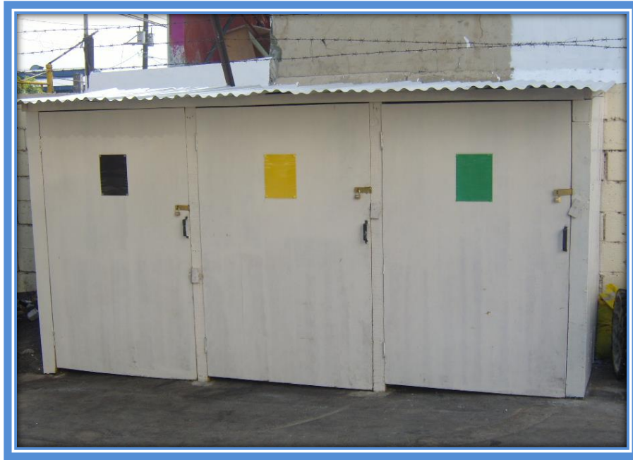
Figure 16- SAH's Temporary Waste Storage Area
