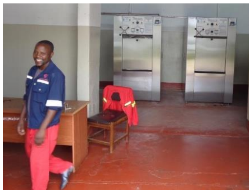
(New autoclaves, installed at Kabwe Regional Hospital, Zambia, 2019)
